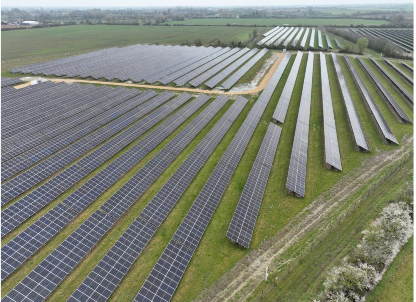
Plate 1: Typical Solar Panels
